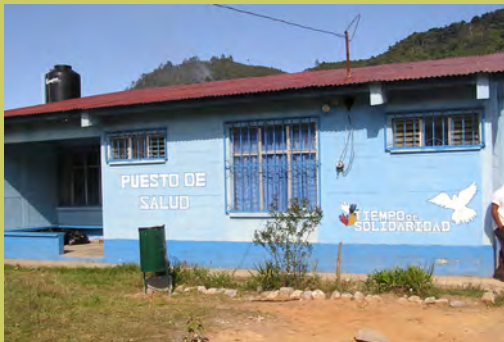
Refurbished Clinic for Cloud Forest
